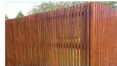
6. Timber slatted external plant enclosure
